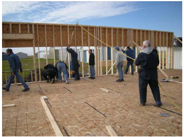
Over 20 volunteers helped secure the walls into position. October 2008
