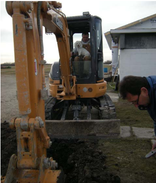
Perry Chromiec, Gil Frechette, Tom Stoyka, Gil Bourrier, Adrian Meilleur and Brian Kirk looking for hot wires feeding The maintenance building and some hangars. Dale Chevalier operating the excavator donated by Darco Ent. with his dog "Buddy"
