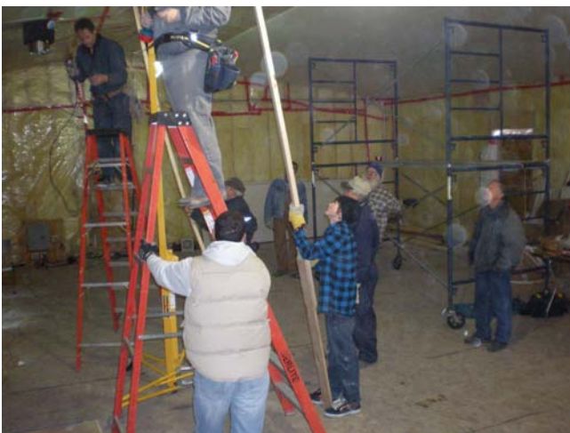
Arie Lazarus, Wilem Pokornik, Al Heim, Bob Hamel, Doug Render, Dale Chevalier, Vic Prefontaine, Gil Bourrier And Dani Pokornik installing drywall. December 2008 to March 2009
