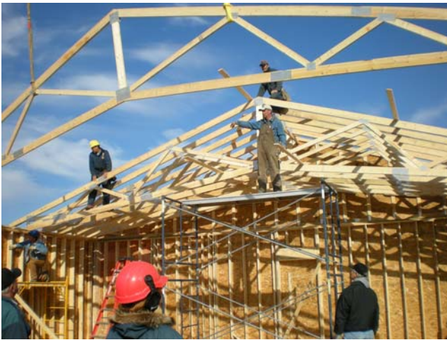
Adrian Meilleur orchestrated the movement of the trusses into place
