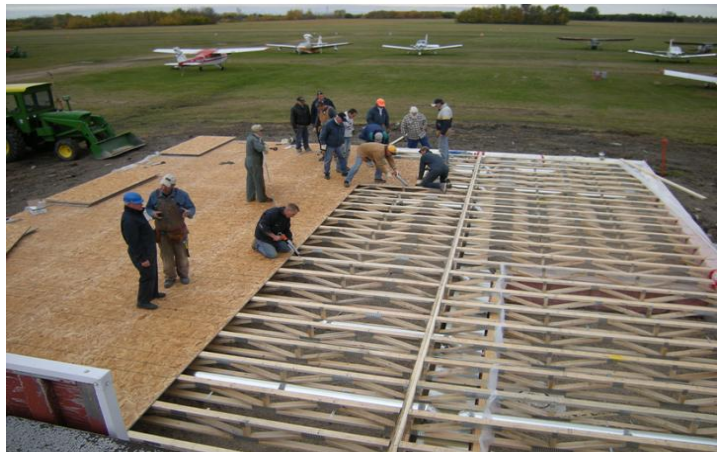
Volunteers laying down the floor, October 2008
