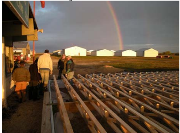
Rainbow at Lyncrest. Wizer Bldg Inc. floor trusses installed
