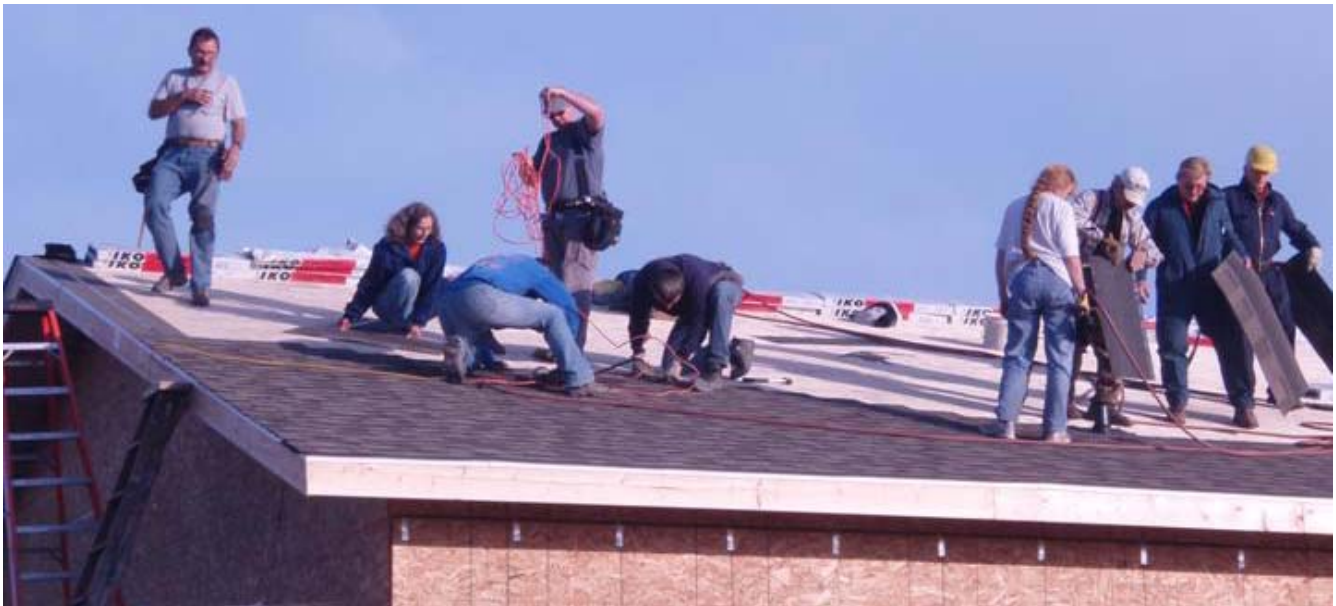
Another crew of volunteers install the shingles. November 2008
