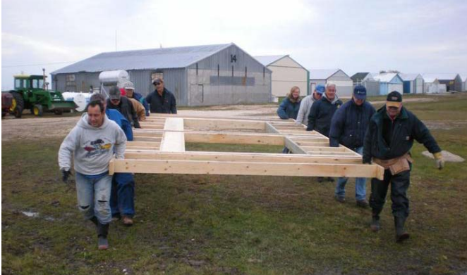
The walls were built in sections were built in sections and Carried into position. October 2008
