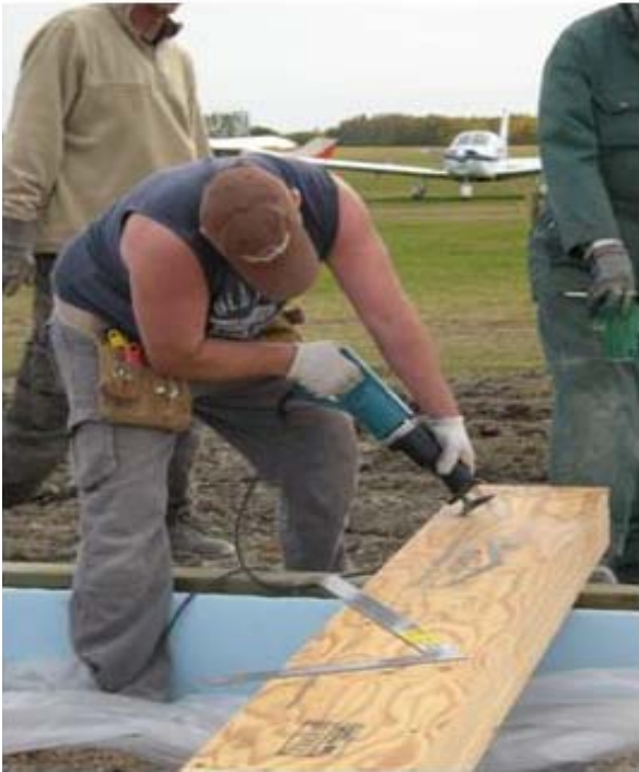
Dani Pokornick cutting off the end of the LVL beam.
