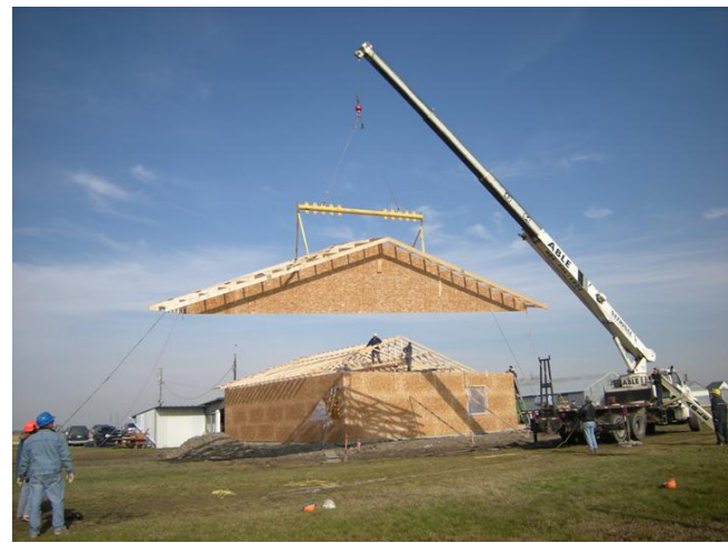
Able Crane donated equipment and an operator to set trusses into position.
